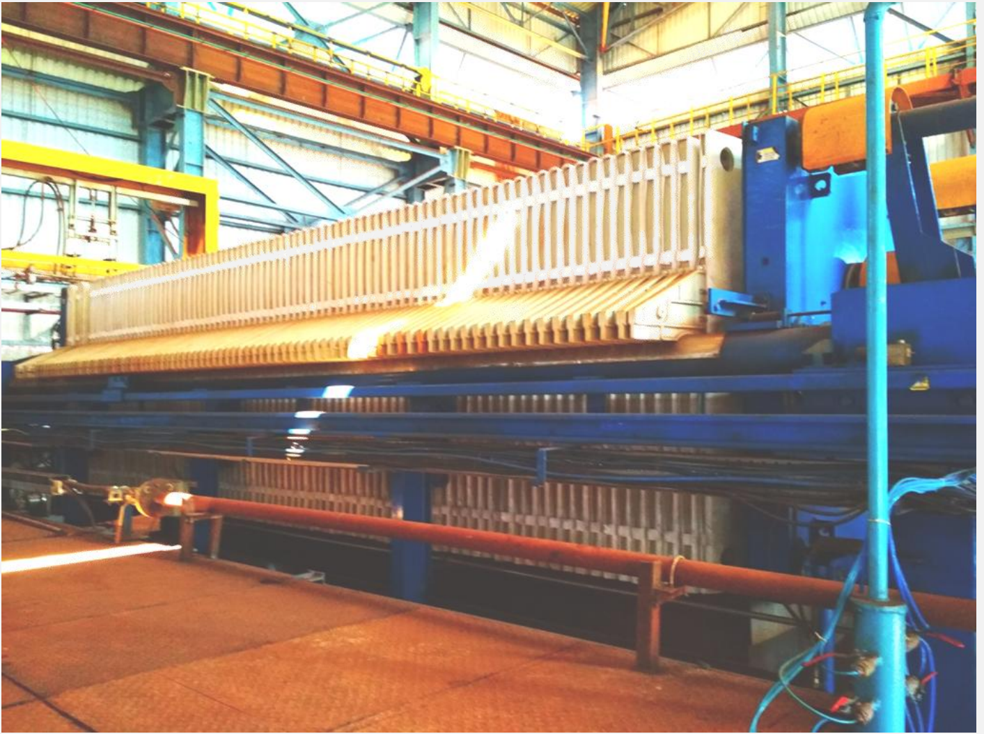
Installation at JSPL Angul for BF – GCP Slurry
